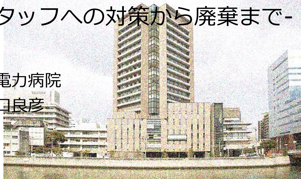
KANSAI ELECTRIC POWER HOSPITAL
